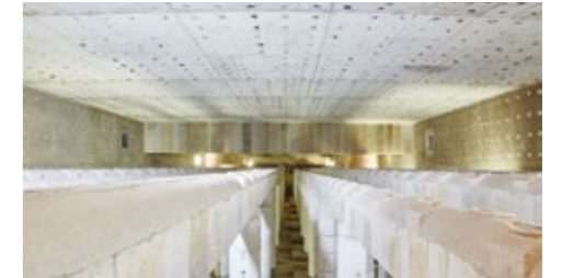
Inside view of the biggest reheating furnace in Europe built by John Cockerill
