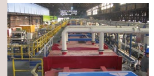
Replacement of chemical section for CPL at ThyssenKrupp, Germany
